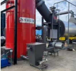
Self-cleaning rotary boiler for solid waste - Horizon +
