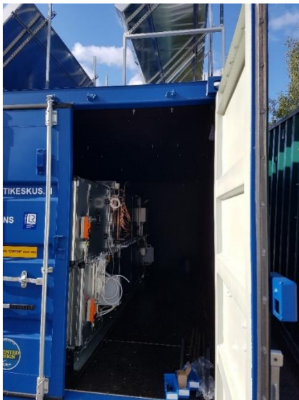
Fig. 2. Air supply unit and integrated heat pump with radiators in the container (left). The other container serves as a drying chamber (right). Biomass can be moved and circulated with a bottom agitator and chain conveyor. Source: VTT
