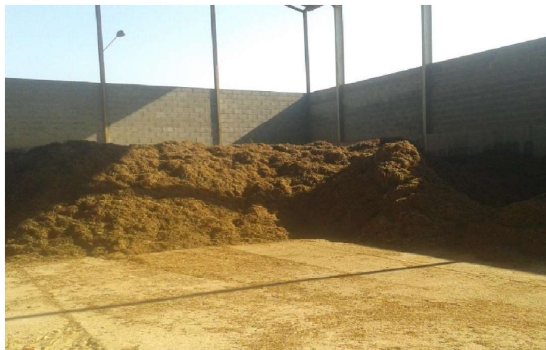
Figure 7: The roofed storage facility (Source: Vineyards4heat).
